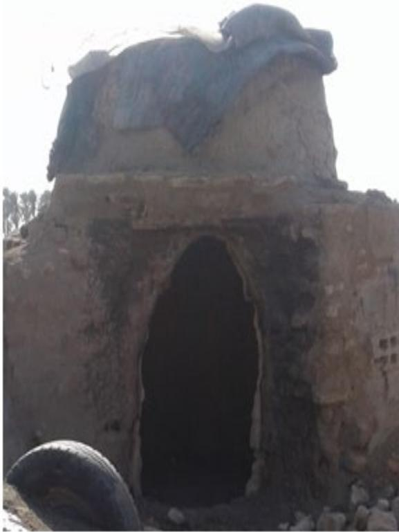
**Picture 4.** The photo depicted by the researcher shows the method of closing the hole, which is used to regulate the position of pots made of clay inside the oven after filling the oven.
